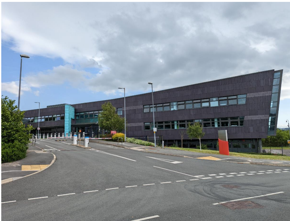
Figure 4.20 Sarn Mynach Offices, Llandudno Junction
