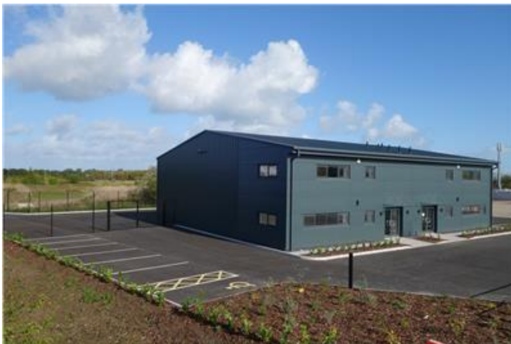
Figure 4.10 Tir Llwyd Industrial Estate, Kinnel Bay
