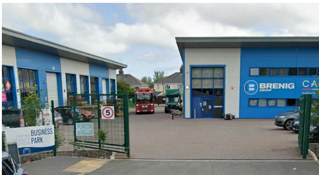
Figure 4.29 Former Dairy Site, Mochdre.
