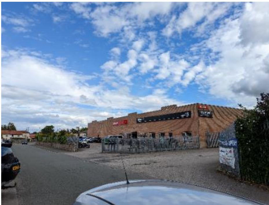
Figure 4.2 Peel Street, Abergele
